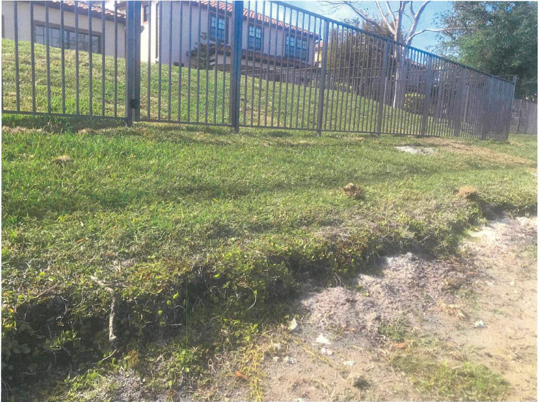
PHOTO #4A: Modified rear yard slope due to pools/deck construction
